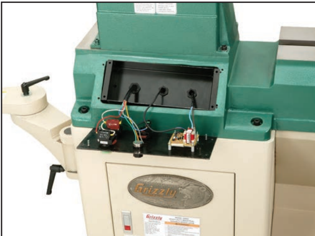
Figure 71. Control panel wiring.
