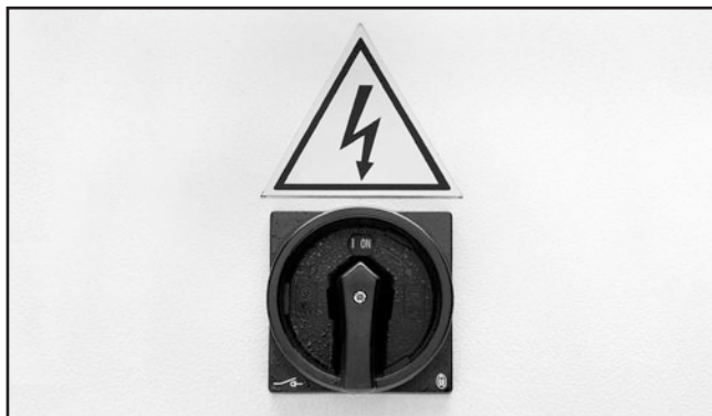
Figure 69. Master power switch.
