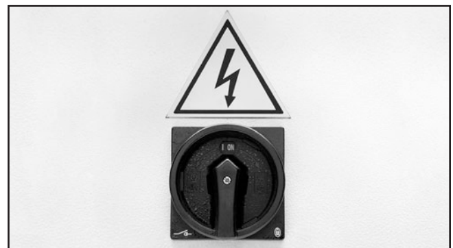
Figure 18. Master power switch in ON position.
